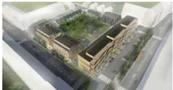
KV KUMMINEN apartments, Orebro, Sweden
